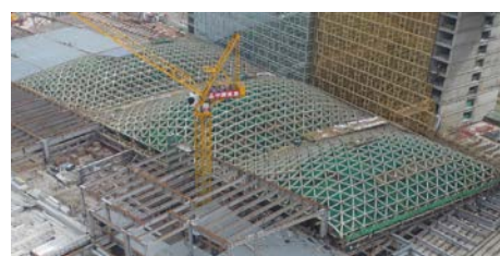
(a) Overall view
