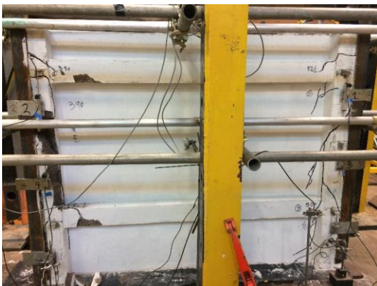
Fig. 9. Failure profile of concrete of specimen T1-LWC.
