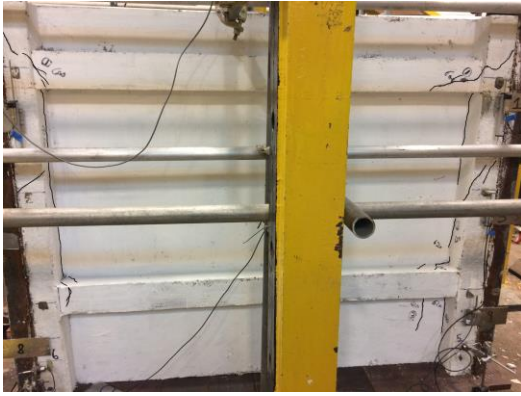
Fig. 8. Failure profile of concrete of specimen T1-NC.
