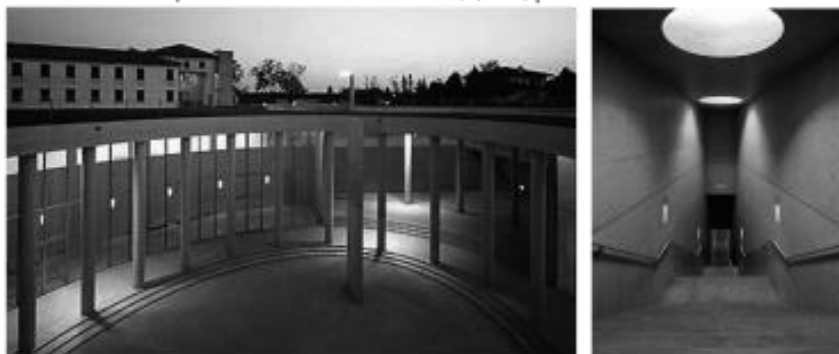
Fabrica Benetton Communication Research Center, (Treviso) | Italia 1992-2000
