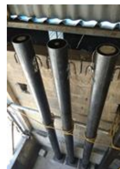
Fig. 3. Concreting of specimens.
