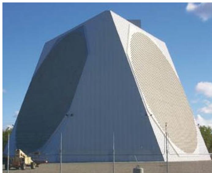
Figura 2.5 Antenas phased array (barrido360°).
