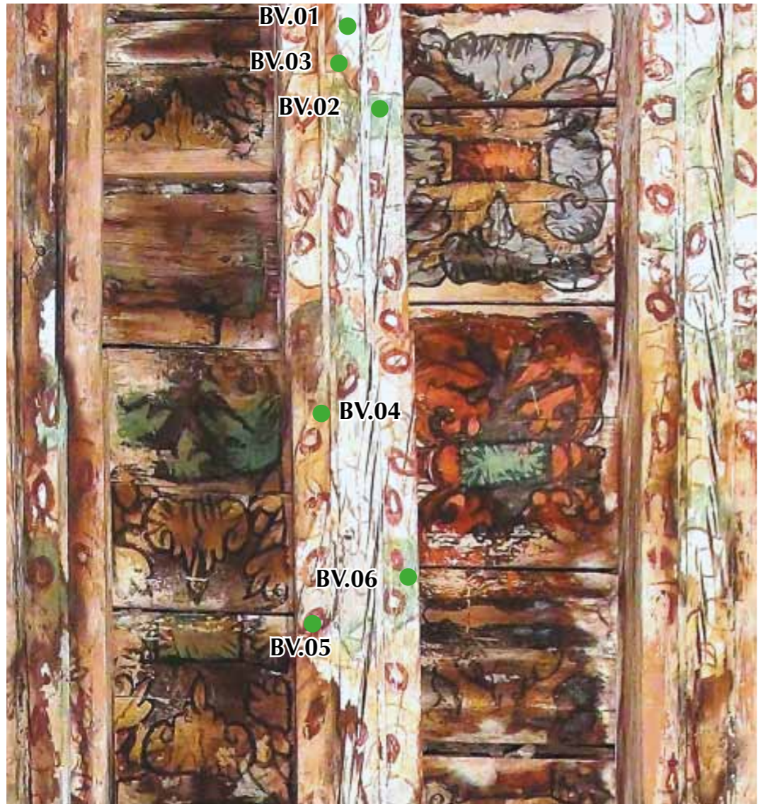
Figure 11:57. Beams marbling sampling documentation. (Performed by: A. Pizarro, P. Ortega & K. Muñoz Alcocer, 2015).
