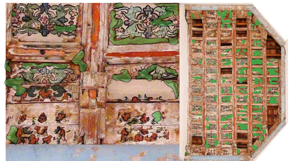
■ Botanic motifs paint losses ■ Marbling paint losses ■ Humidity stain
