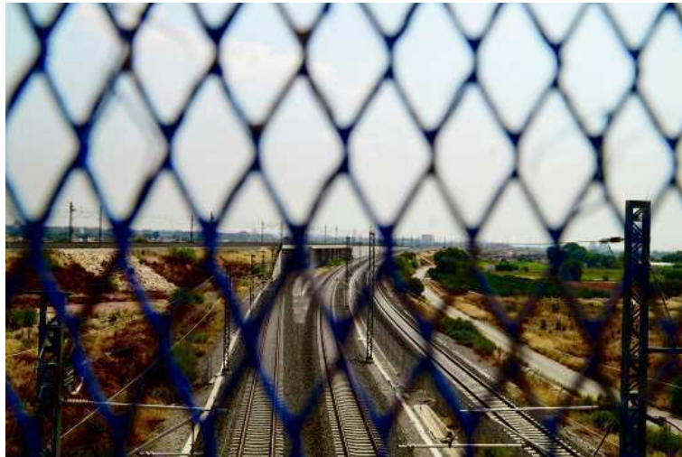
Figure 2. High Speed Train infrastructure seen from the bridge to pass.
