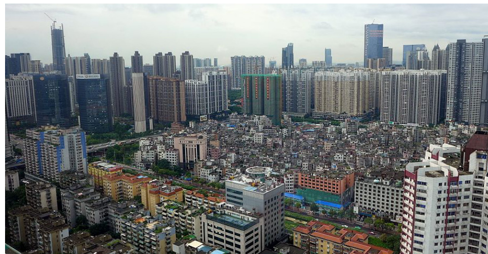
Figure 1. View of Xian village, Guangzhou, China. Source: web.
