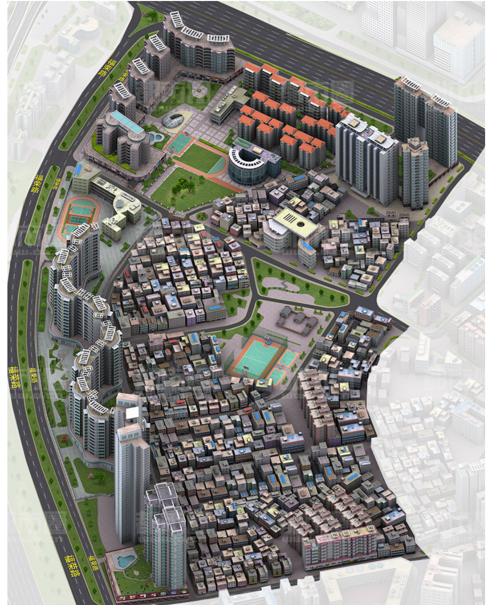
Figure 83. Aerial view of Xiasha village. Source: http://china.earthol.com/bd/sz/
