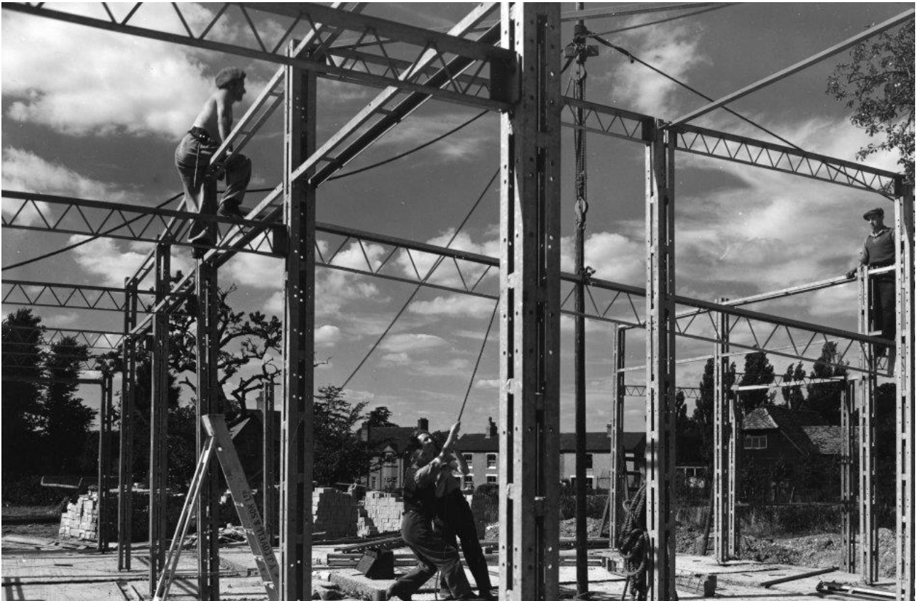
Figura 74. Estructura de la Primary school, Leavesden.
