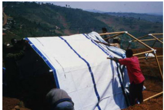
Figura 2.10 Paper Tube Emergency Shelter
