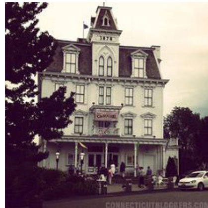
Fig 14. Goodspeed Opera House
