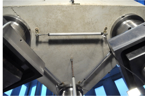
CARA INF – Colapso
