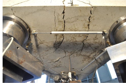
CARA INF – Colapso
