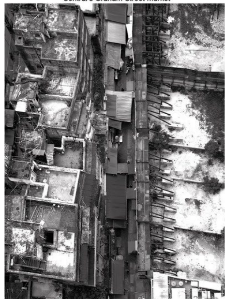
4. Graham Street, Central: current condition with open-air wet market, urban block on right demolished.
