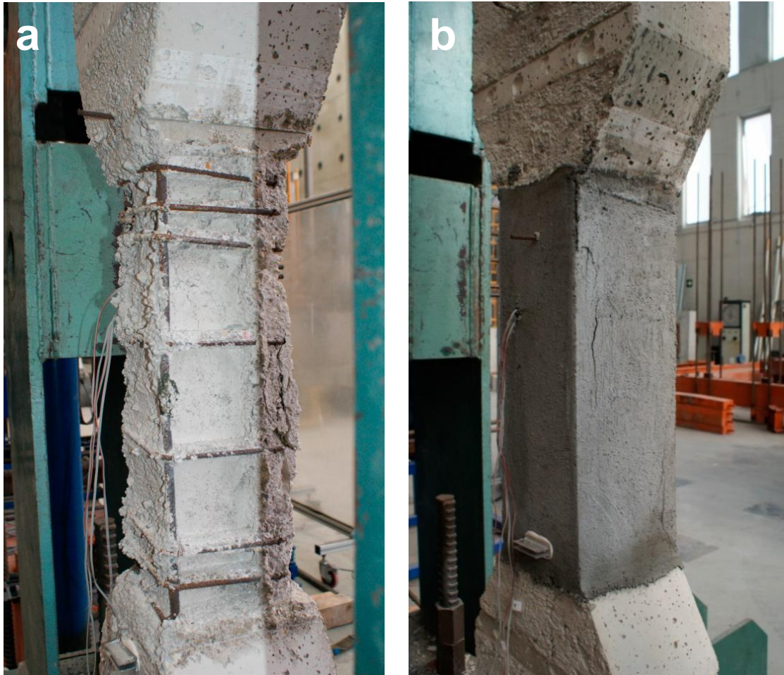
Fig. 5. a) Damaged column (DC); b) Failure mode: Specimen R3B (repaired column with Class R3 mortar with bonding agent).
