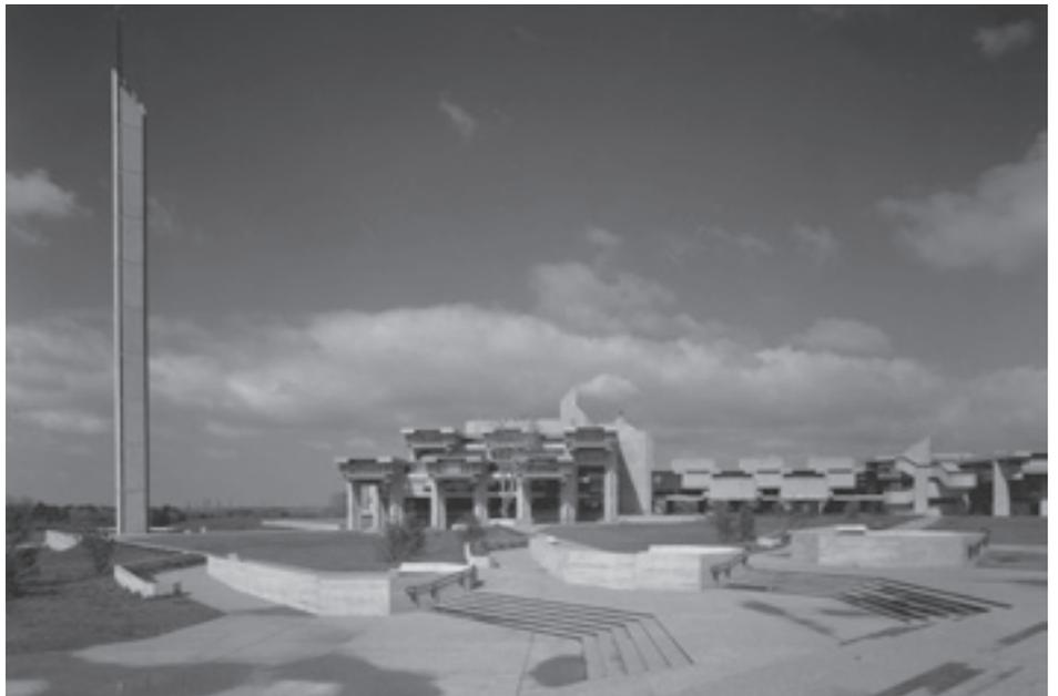
the campus is through a road that connects to the circular ring and parking which is camouflaged by vegetation. The topography was modified to generate different platforms that in a centrifugal way lead to the faculties but come together in a space representative of the union conceived as an outdoor amphitheatre. Its construction was carried out in several phases but developed as a whole. The volumes are fragmented by sections to enrich the visuals and avoid monotony [fig. 3 and 4].
