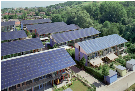
Figure/ Figura 2. 55 Solar panels in residential buildings [ www.habitatdurable.ch ]
