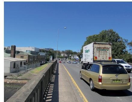
Canal Rd, bridge
