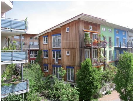
Figure/ Figura 2. 54 Vauban apartments [ www.maires88.asso.fr ]
