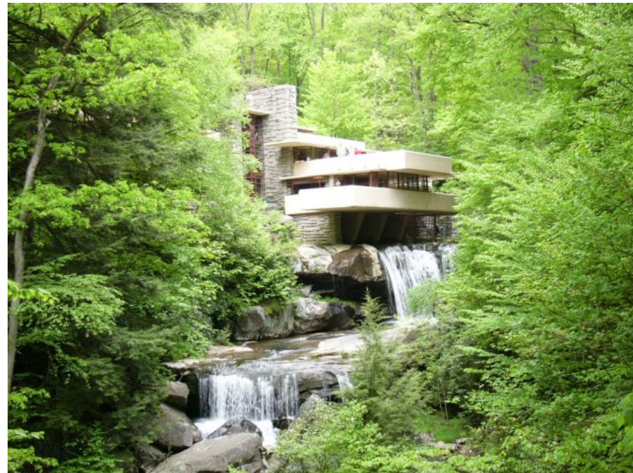
Fallingwater de Frank Lloyd Wright (Pennsylvania) (2.15)
