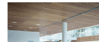
T.5-T.6_HUNTER DOUGLAS SISTEMA GRID MADERA +12,10-12,40m
