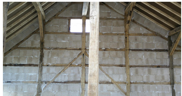
Figure 3 Insulation using hempcrete blocks for a half-timbered farmhouse (iso hemp.com)
