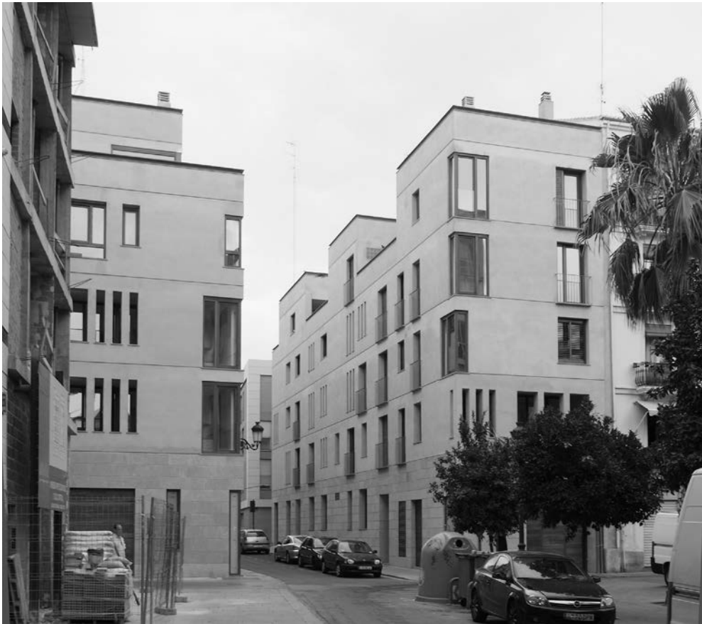
Figure 9. Recaredo building. View of buildings A (left) and B (right) onto Roger de Flor Street. Building B shows in perspective the result of the “crenellation” and the studied distribution of windows seeking to break up the horizontal reading. (Photo by Tato Herrero, 2010)
