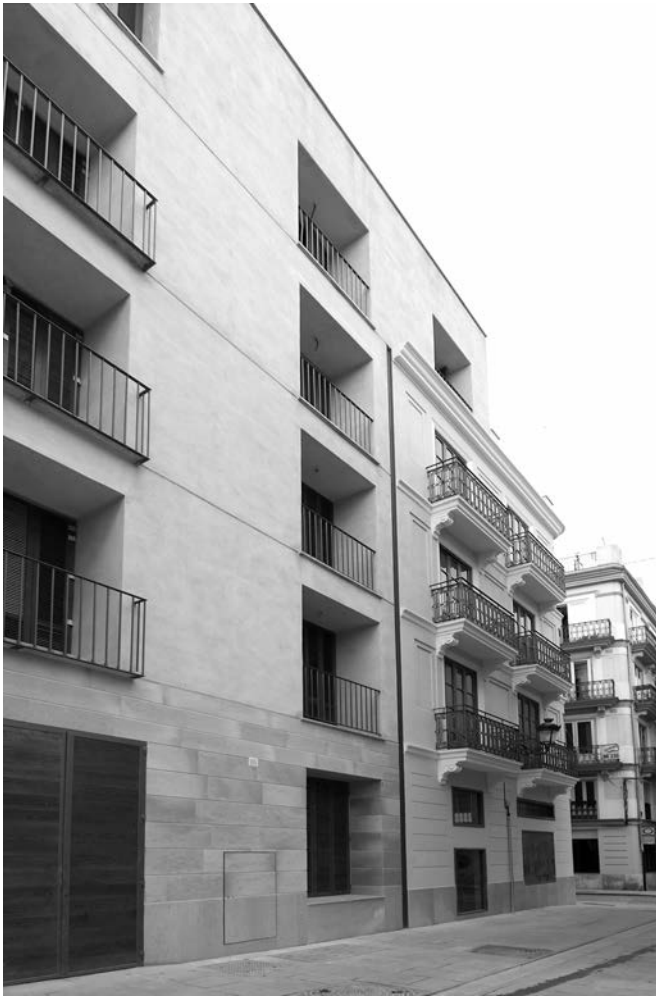
Figure 4. Maldonado building. Detail of the new thick façade overlapping the reconstruction of the historic façade in order to show this contradiction. (Photo by Tato Herrero, 2010)
