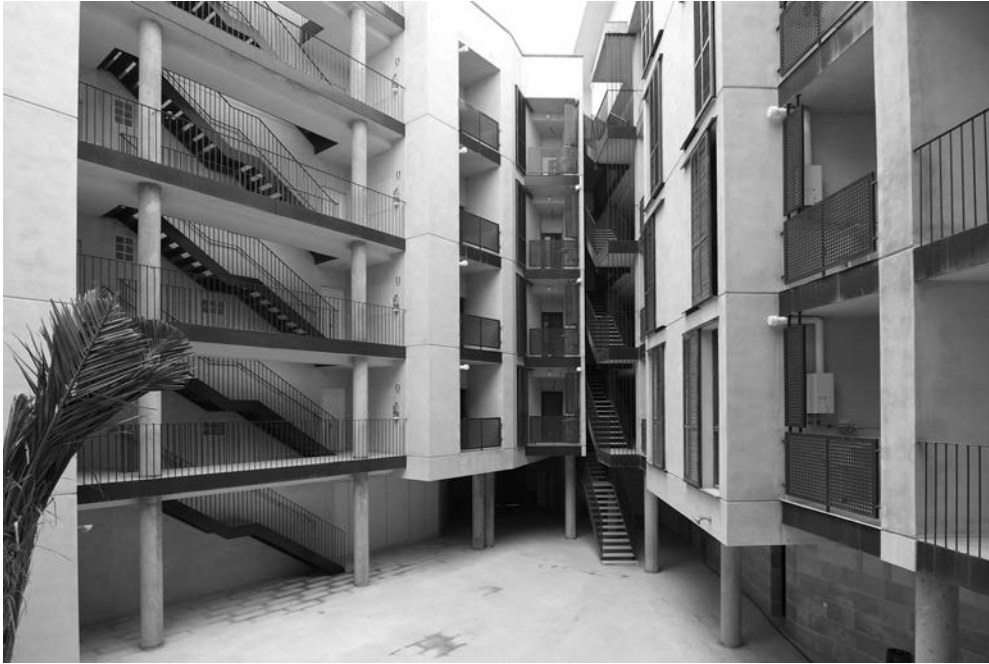
Figure 5. Maldonado building. Partial view of the courtyard with the inner façades opening out onto it, as the center of the life of the building. (Photo by Tato Herrero, 2010)
