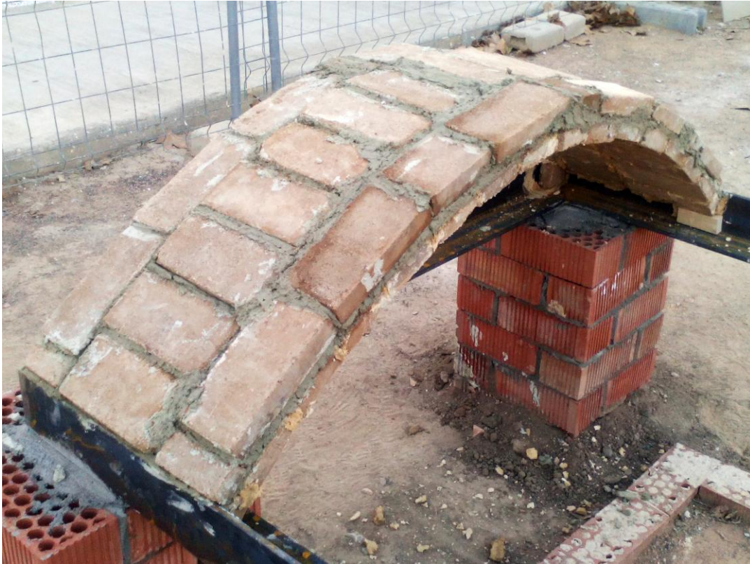
Figure 3. Life-sized model of the tile vaults designed for the school of Baasneere
