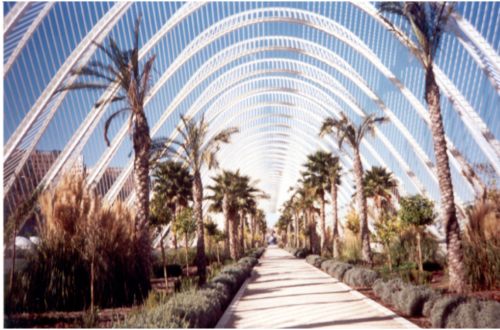
F244. Tramo XI Interior Umbracle A
