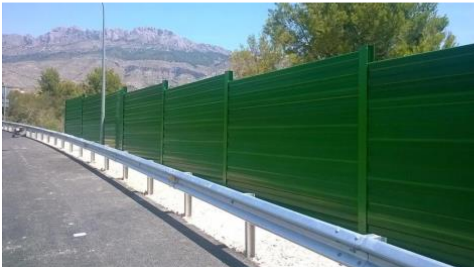
Illustration 23- Example of acoustic screens
