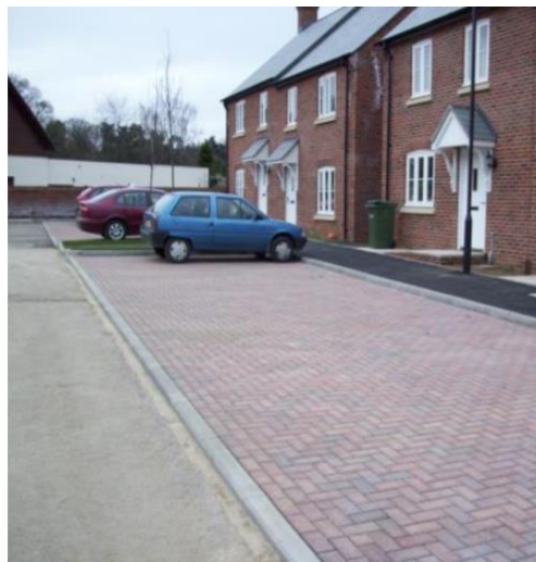
Figure 3. Permeable pavements. Source Susdrain
