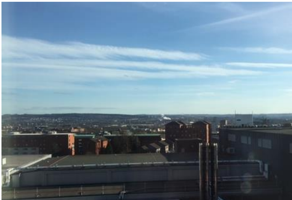
Figure 21. Roof of the library building
