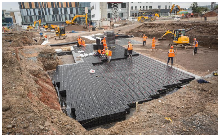
Figure 5. Geocellular systems. Source: Projectscot
