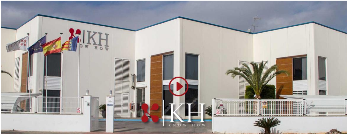
Figura 3. Nave industrial KH Vives.
