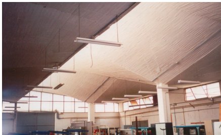
Figure 4. Interior view of the original building
