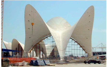
Figure 8. Cover of the access building under construction.
