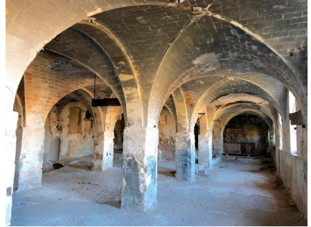
Figure 3. Ground floor of 20 palm vaults in Solers factory.
