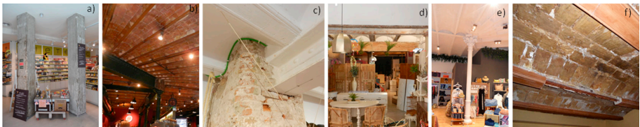
Figure 8. Uncovered structural elements. Source: the authors (2017).
