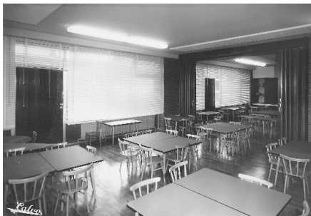
Figure 3. View of the patio area and interior of the classrooms. Source: Llado, A. (1996) Navarro, Pablo (1959).
