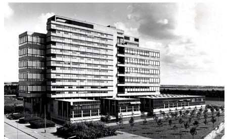
Figure 1. New Faculty of Architecture by van der Broek & Bakema Architects Community (1970). Source: www. Broek&Bakema.nl .
