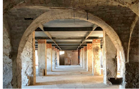
Figure 5. View of the renewed enguilat grid system.
