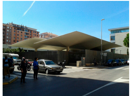
Figure 5. Exterior view of the renovated building.
