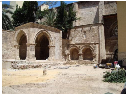
Figure 58. Conservation condition of San Juan, 2017.
