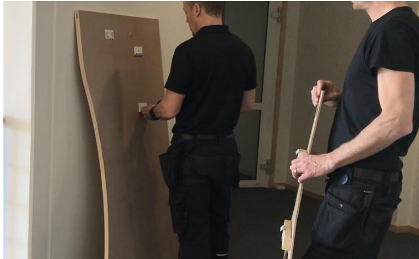
Figure 74. Mounting test hangers-system.
