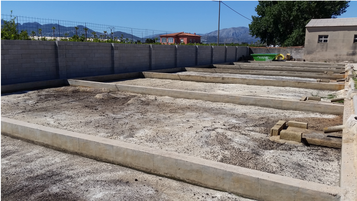
Figure 13: Side view of the sludge drying basins within the WWTP site.
