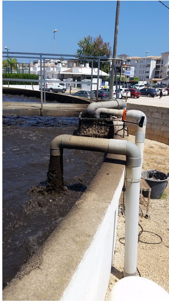
Figure 42: Another view of the Kestrel mobile meteorological weather station along with an active outflow of the canalization and the sludge recirculation into the bioreactor.
