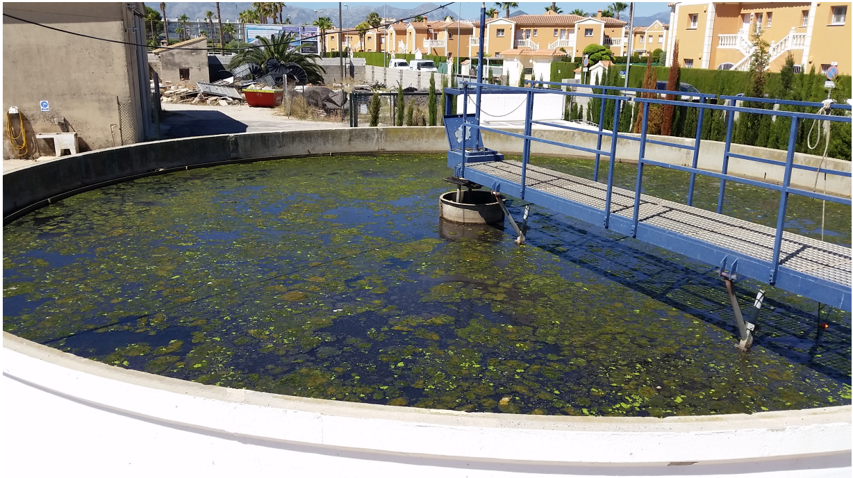
Figure 11: Photograph of the decanter next to the bioreactor within the WWTP site on 20 June 2018. The process of surface sludge building can be observed when comparing this picture to photograph 12 taken more than one month later on 27 July 2018.
