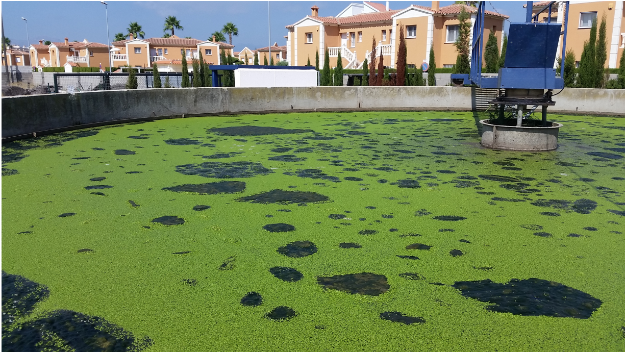
Figure 12: Another photograph of the decanter more than one month later than picture 11 showing the difference in surface sludge building. For this reason, the surface sludge is pumped off just like the thicker bottom sludge of the decanter.
