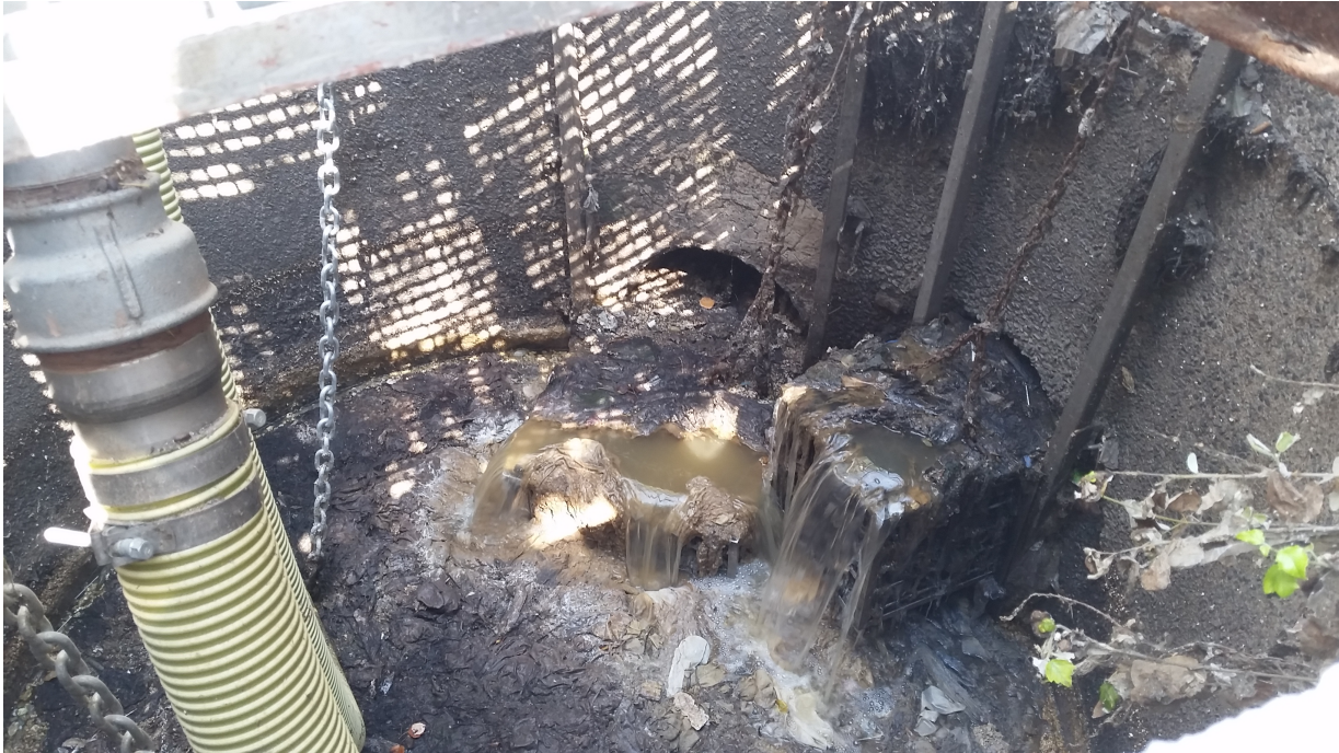
Figure 15: View inside the well of Pumping Station 2.
