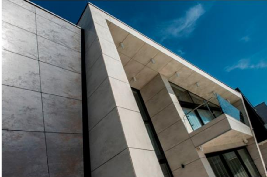
Figure 6: Ventiladed façade in a unifamilial building in Prishtina (Kosovo). [Online] Available: https://www.grespania.com
