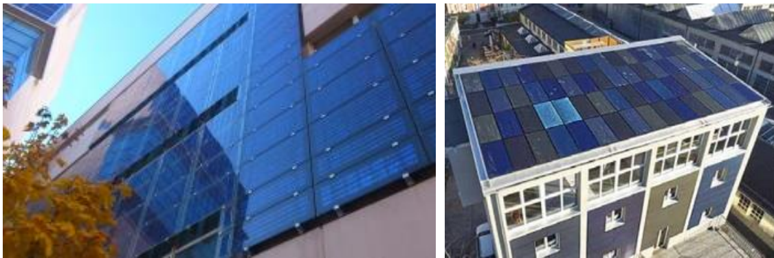
Figure 7: BIPV's installed in the façade of a building (left) and in a rooftop (right). [Online] Available: https://www.glassonweb.com (left image), https://www.skoltech.ru (right image).
