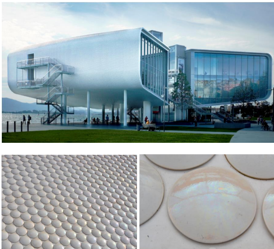
Figure 5: Top images shows the headquarters of the Botín Foundation in Santander (Spain). Bottom images show ceramic tiles which cover the façade and roof of the headquarters. From: "Iridescent Techniques in Ceramics: Physico-Chemical Analysis and Colorimetric Characterization of the Headquarters of the Botín Foundation in Santander" by Víctor Echarri-Iribarren et. al., Appl. Sci. 2019, 9, 1521.
