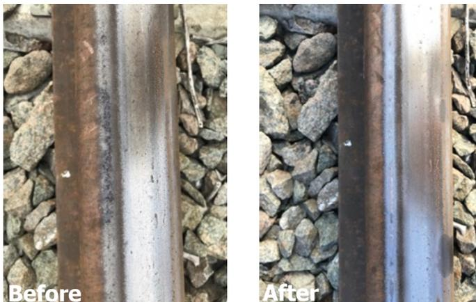
**Fig. 13.** Effect on railhead oxidation
