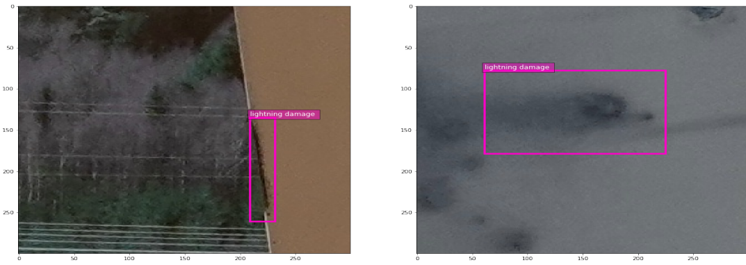
Figure B.9: Lightning damage
