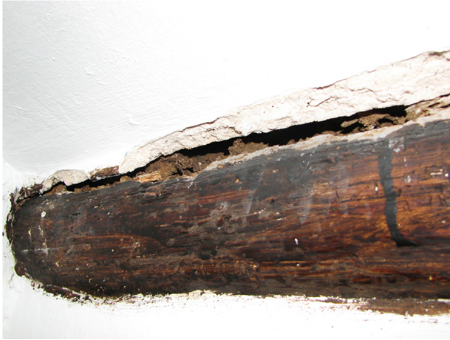
Figure 10. Degradation of the surface between the timber and the vaults caused by wood boring insects (Marquees of Benicarló's Palace, Benicarló, Castellón de la Plana)
