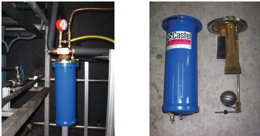
Figure 3.5: Oil separator (left), unmounted oil separator (right)
