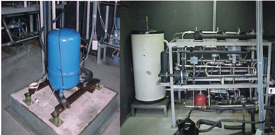
Figure 3.2: Compressor (left), condensation unit (right)
