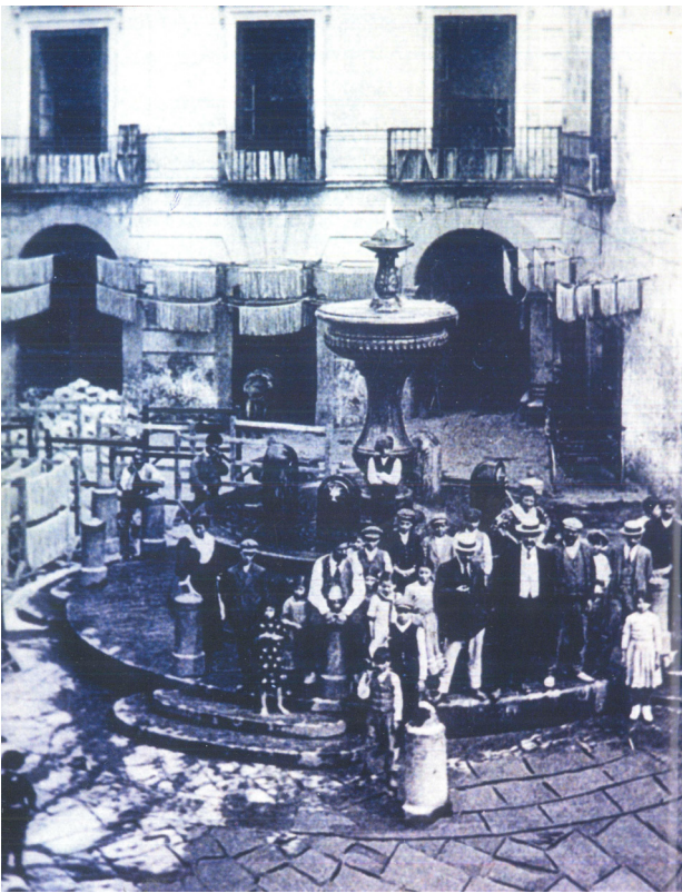
Figure 2. Fountain of Piazza Trivione.
