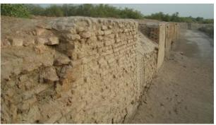
Fig. 3 The brick are being attached by the salted water from the back, of the inclining wall
