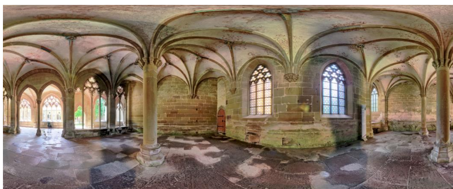
Figure 60. HDR image from the new scans.
