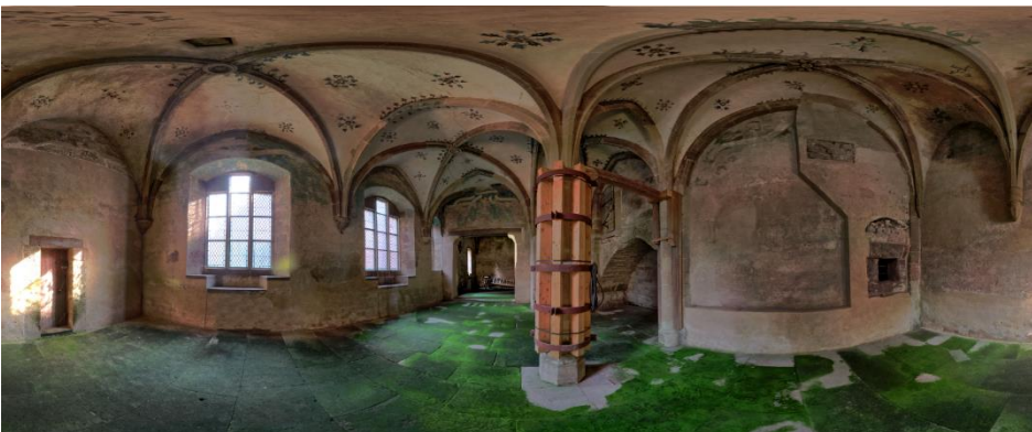
Figure 53. Image from the new scans.
