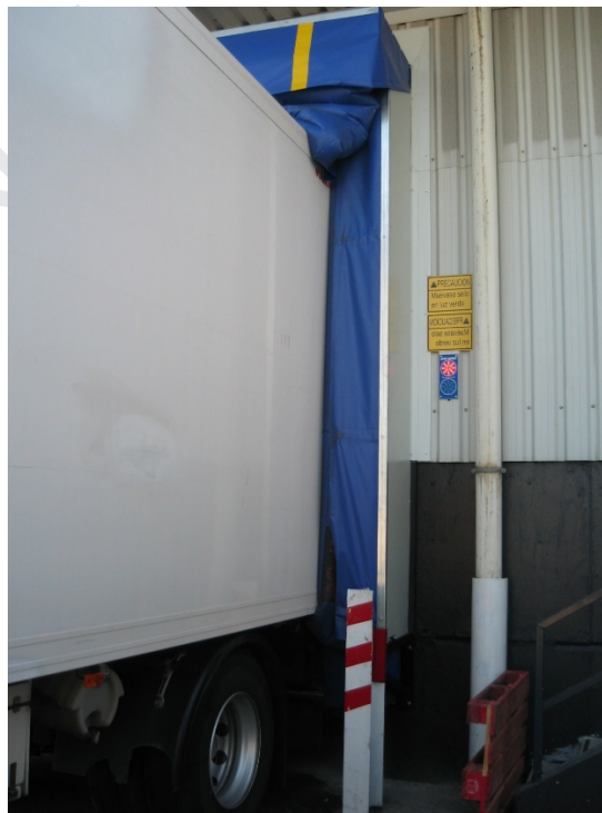
Figure 2: Exterior view of inflatable dock adjusted to the truck shape.
