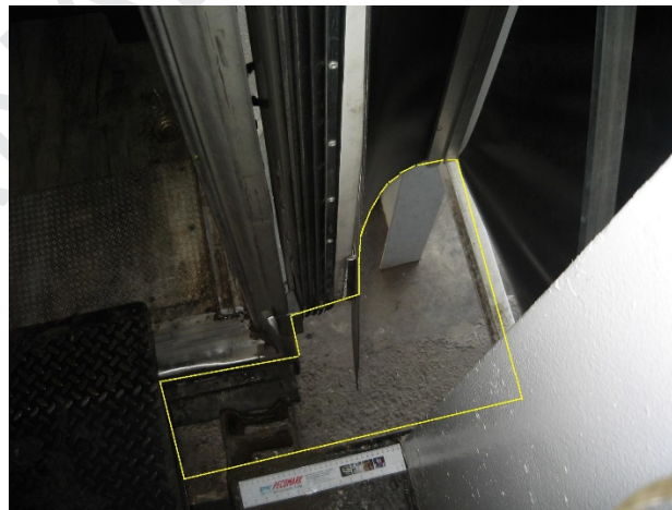
Figure 5: Main openings in a simple flaps dock door shelter
