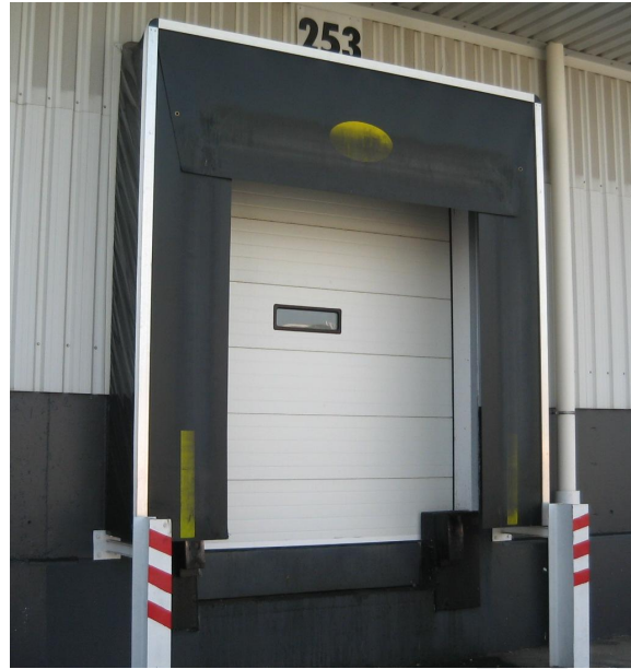
Figure 1: Exterior view of simple flaps dock
