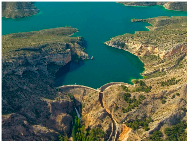
Figure 2. Aerial view of Cueva Foradada dam and its fixed crest spillway.
