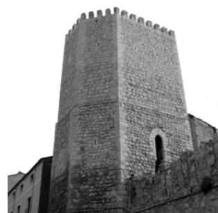
A TORRE BOMBARDERA
