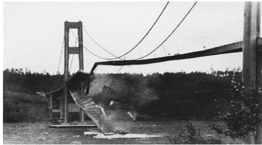
Figure 1-1. Tacoma Bridge in US (1940).
