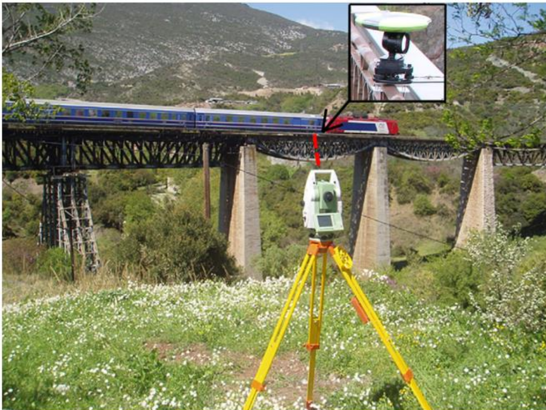
Figure 2-3. Gorgopotamos Railway Bridge and the robotic total station in the foreground.
