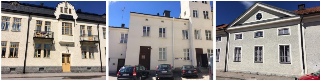
Fig. 15: Examples of real buildings in Arboga similar to category 3. Photo: Johan Torgén [22]
