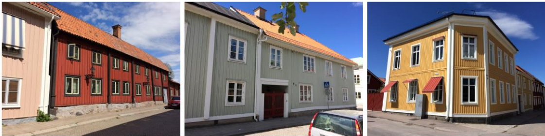
Fig. 13: Examples of real buildings in Arboga similar to category 2. Photo: Johan Torgén [22]
