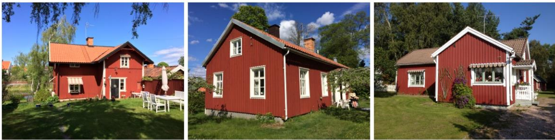
Fig. 17: Examples of real buildings in Arboga similar to category 4. Photo: Johan Torgén [22]
