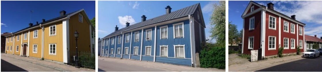
Fig. 11: Architectural examples of category 1 buildings. Foto: Johan Torgén [22]
