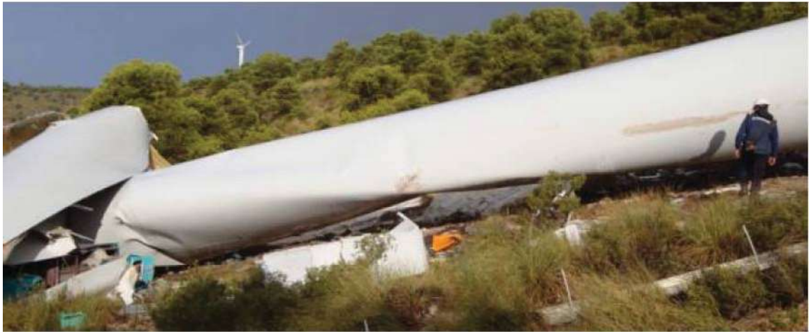
Fig. 3. View of the tower the day after collapsing
