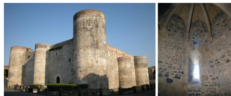
Fig. 7. Ursino Castle: angular view of the external facades and space covered by cross vault on corbels ( http://www.icastelli.it/it/sicilia/catania/catania/castello-ursino-o-svevo-di-catania ).
