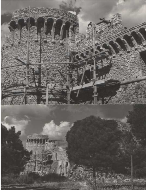
Fig. 8. Recovering works on the castle (1962, Photo credits Ing. T.L. Orlandi, from Di Domenico, 2002).
