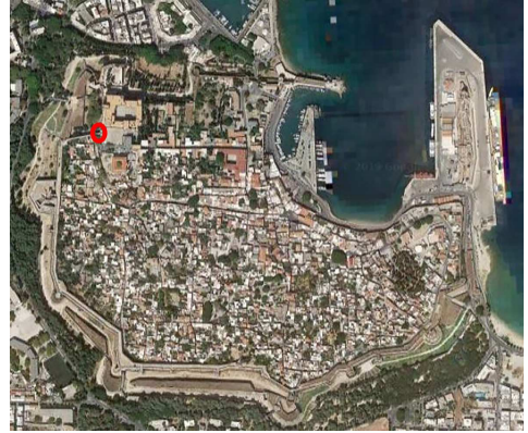
Fig. 4. Aerial view of the Castle of Rhodes (Google Earth).
