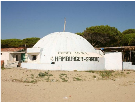
Fig. 4. Transformation of a bunker into a cafeteria (Adnan Asllani, 2005 in Flickr).
