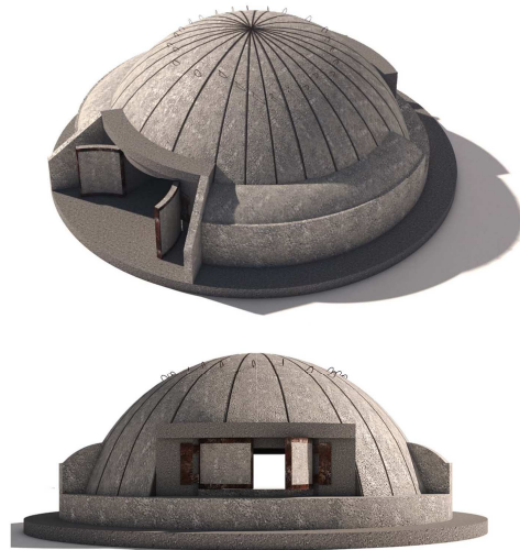
Fig. 2. Reconstruction based on survey documentation. Typical medium size bunker (visualisation Flavio Derivishi & Uendi Konduri, 2019).
