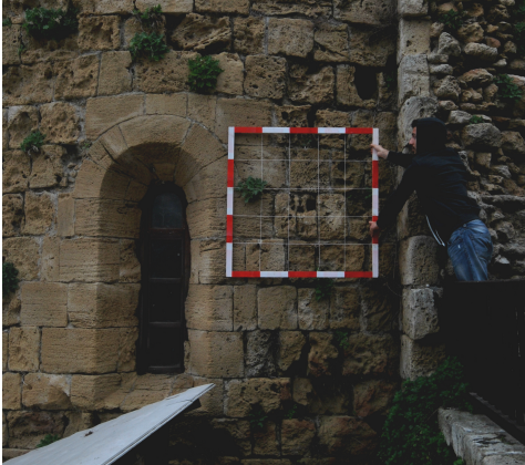
Fig. 4. Survey of the masonry type.
