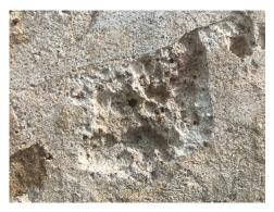
Fig. 10. Plaster mortar from west side of tower wall.
