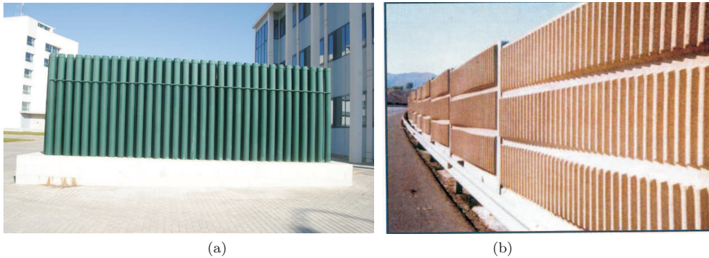
Fig. 2: (a) SC used as acoustic barrier; (b) Classical acoustic barrier.
